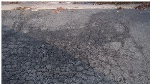
Pavement Condition 11 - 40 (Very Poor/Serious)
