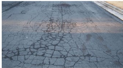
Pavement Condition 11 - 40 (Very Poor/Serious)
