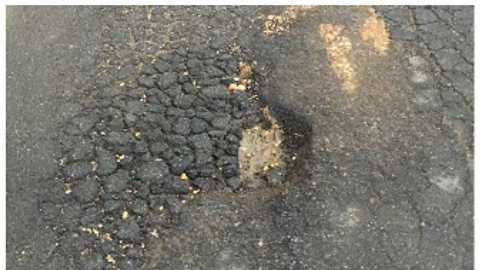
Pavement Condition 0 - 10 (Failed)
