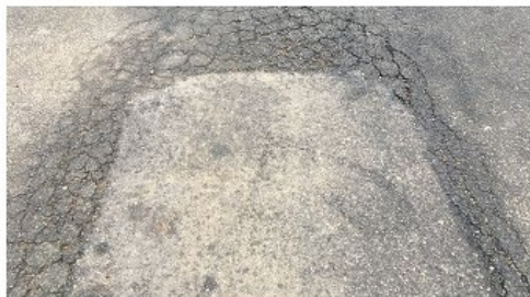
Pavement Condition 0 - 10 (Failed)
