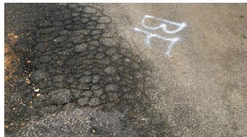
Pavement Condition 0 - 10 (Failed)
