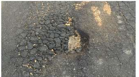
Pavement Condition 0 - 10 (Failed)
