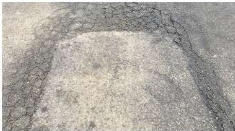
Pavement Condition 0 - 10 (Failed)
