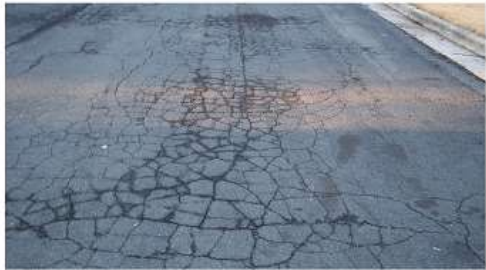
Pavement Condition 11 - 40 (Very Poor/Serious)
