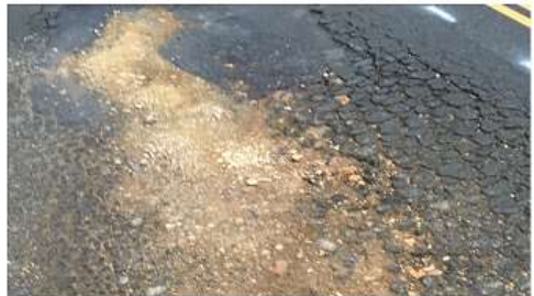
Pavement Condition 0 - 10 (Failed)
