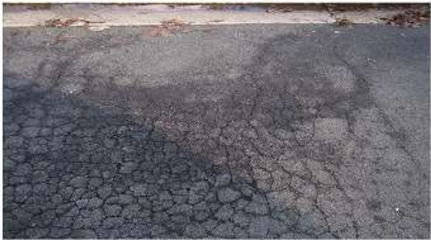
Pavement Condition 11 - 40 (Very Poor/Serious)
