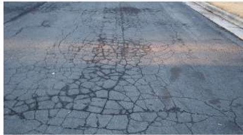
Pavement Condition 11 - 40 (Very Poor/Serious)
