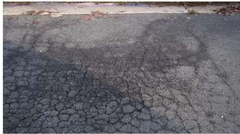
Pavement Condition 11 - 40 (Very Poor/Serious)
