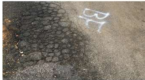
Pavement Condition 0 - 10 (Failed)
