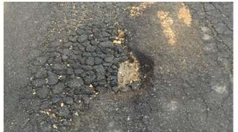
Pavement Condition 0 - 10 (Failed)
