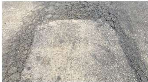
Pavement Condition 0 - 10 (Failed)
