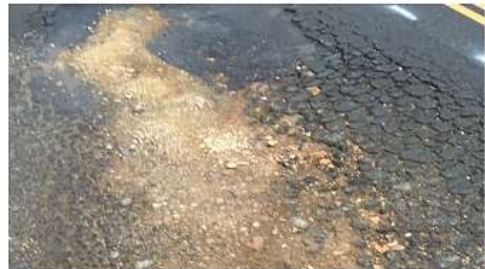
Pavement Condition 0 - 10 (Failed)
