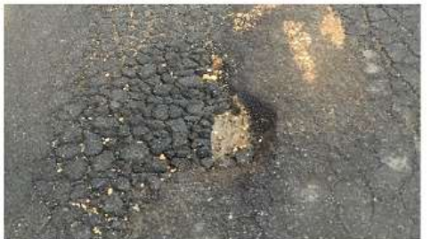
Pavement Condition 0 - 10 (Failed)
