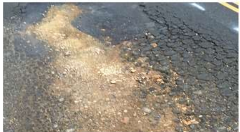
Pavement Condition 0 - 10 (Failed)
