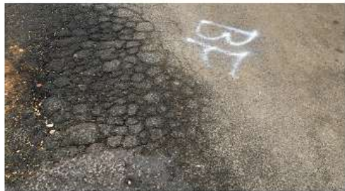
Pavement Condition 0 - 10 (Failed)
