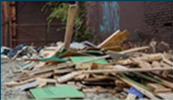
Building Code Violations
